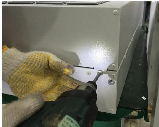
Figure 15: Twist off the screw on the top of the cover
